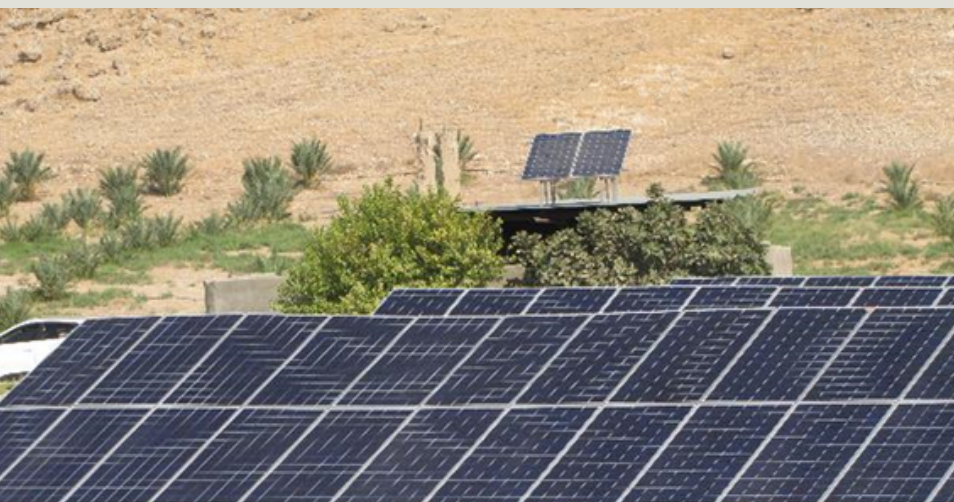
Solar Panels Installation by ESDC
